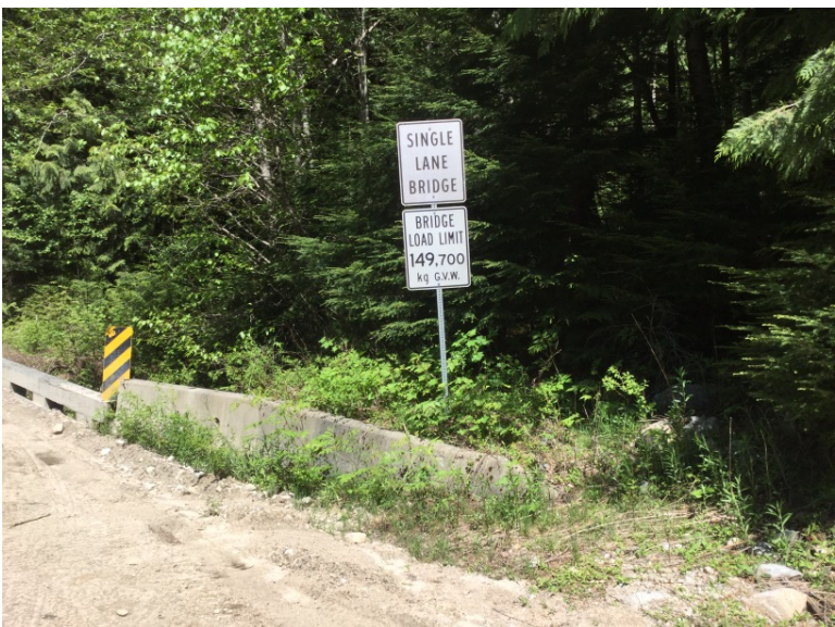
Load Rating Sign
