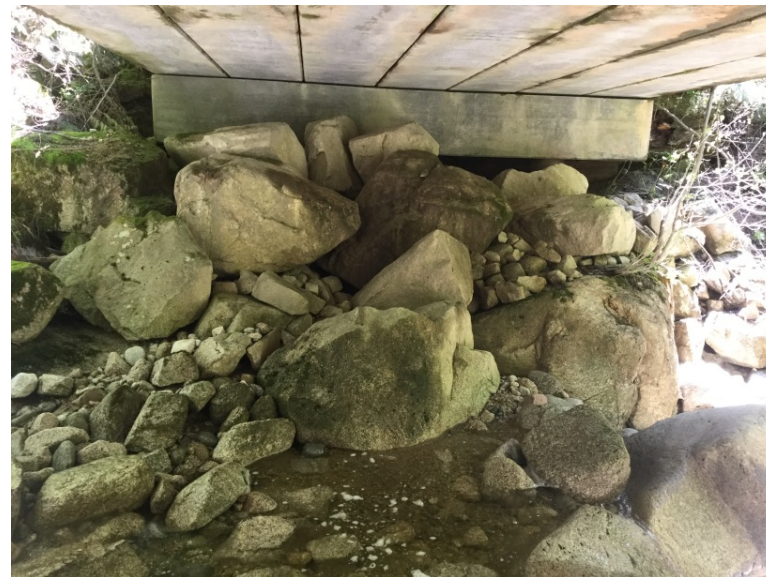
Left Bank Abutment when facing downstream
