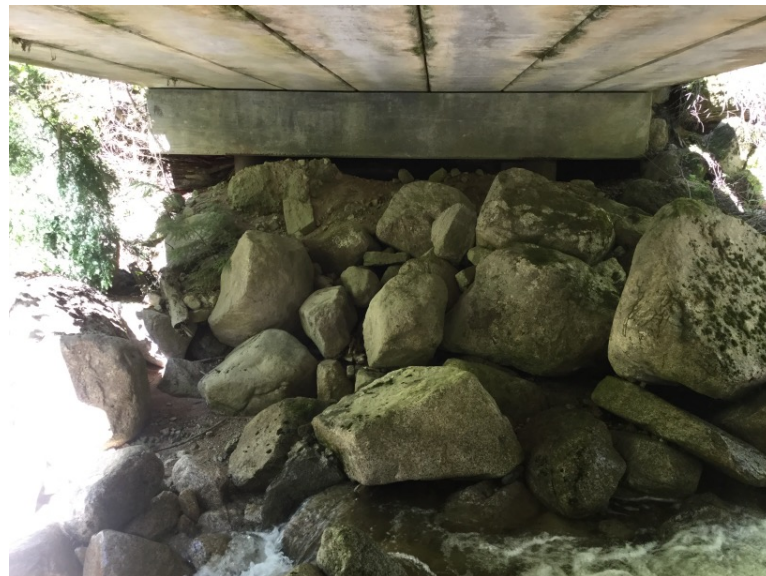
Right Bank Abutment when facing downstream
